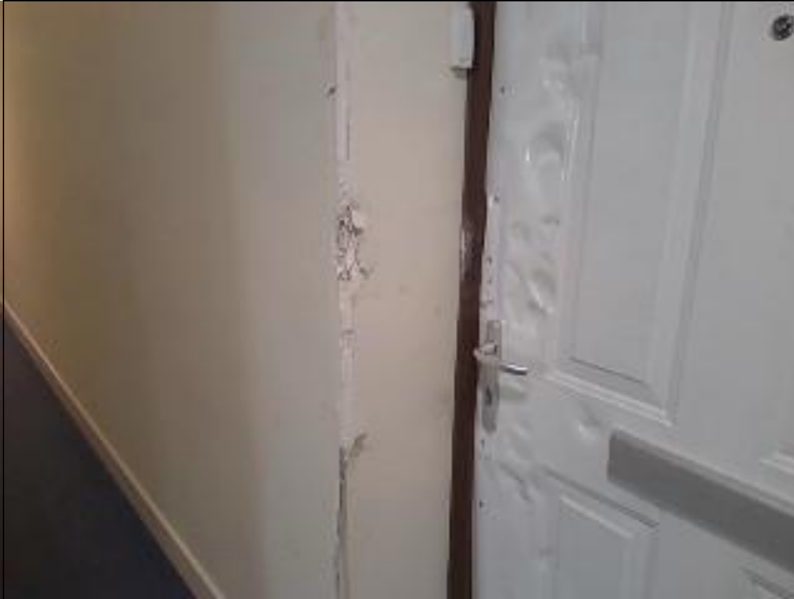
25812_Action_The following fire doors are damag_14
