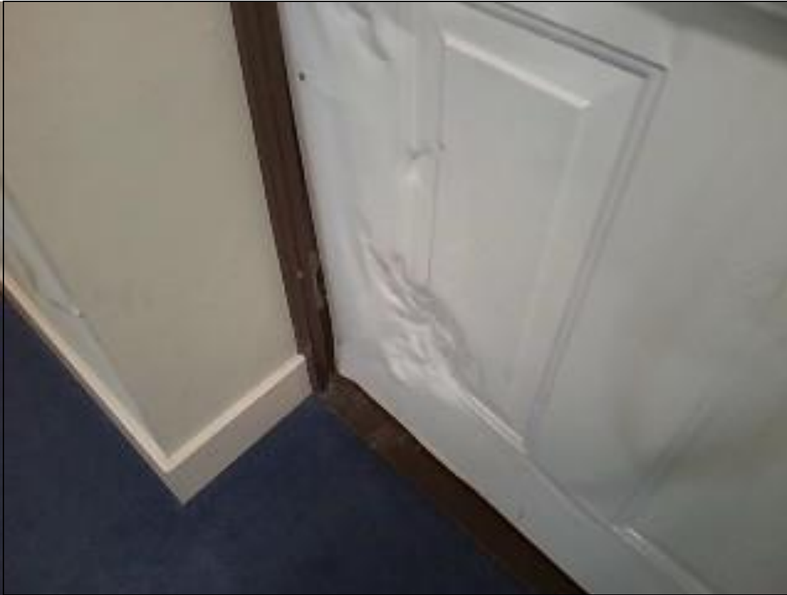
25812_Action_The following fire doors are damag_14
