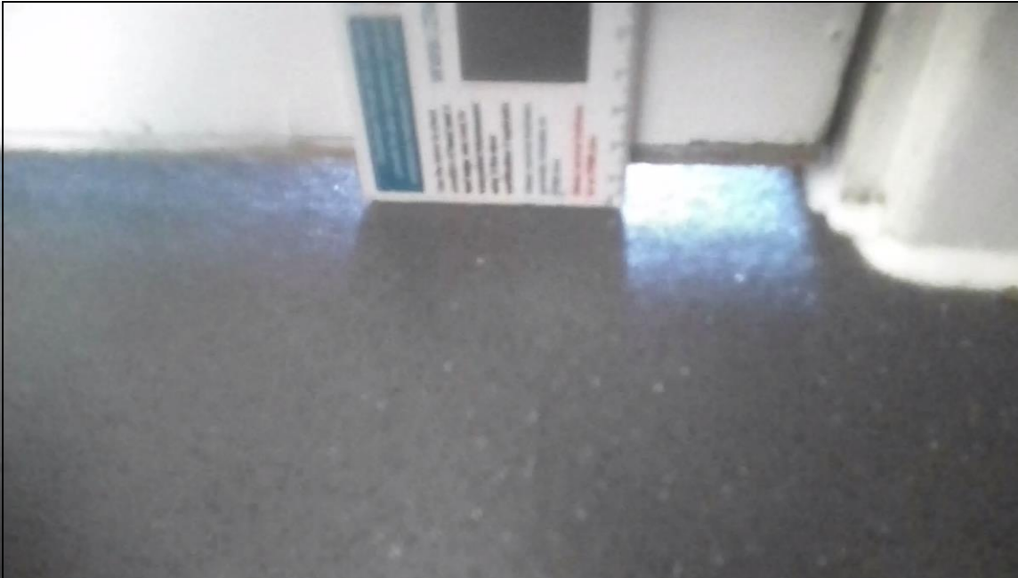
23030_Action_The following doors require mainte_05
